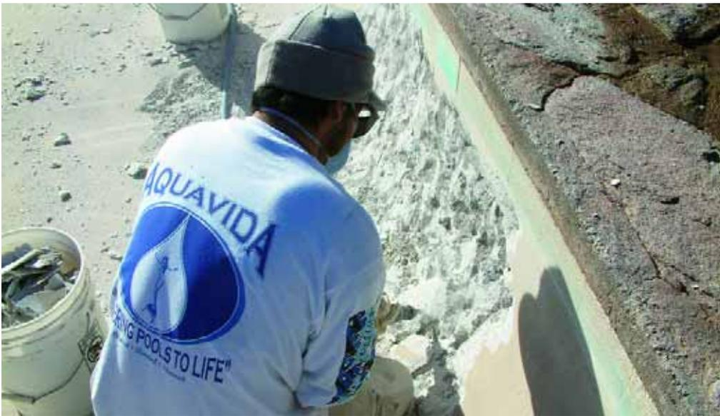
Our first day on site saw us chip out the old plaster finish – a process that clearly had everyone on edge in fear of any collateral damage that might occur with the decks or anything else having to do with the setting. But all went well, and we found that the concrete shell was in great shape and plenty hard enough to put up with our hammering.
